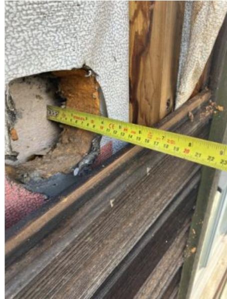
Polyisocyanurate (PIR) in Timber Facade
