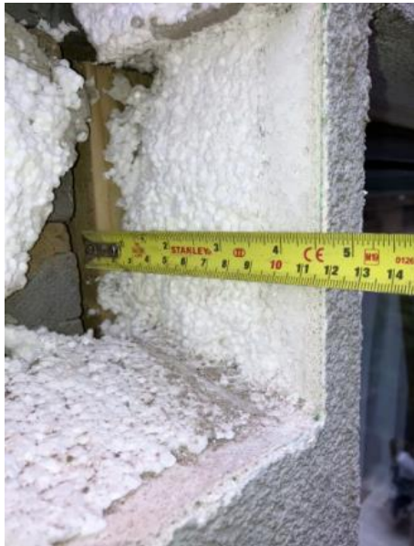
Expanded Polystyrene Styrofoam (EPS) in Render Facade
