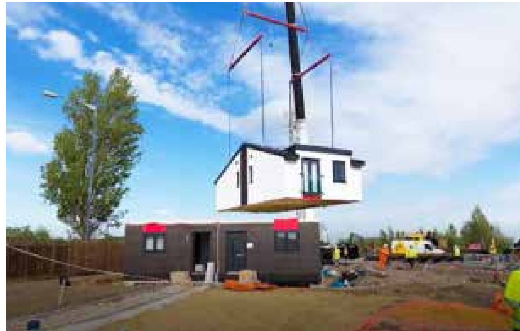
Lifting of volumetric modules
